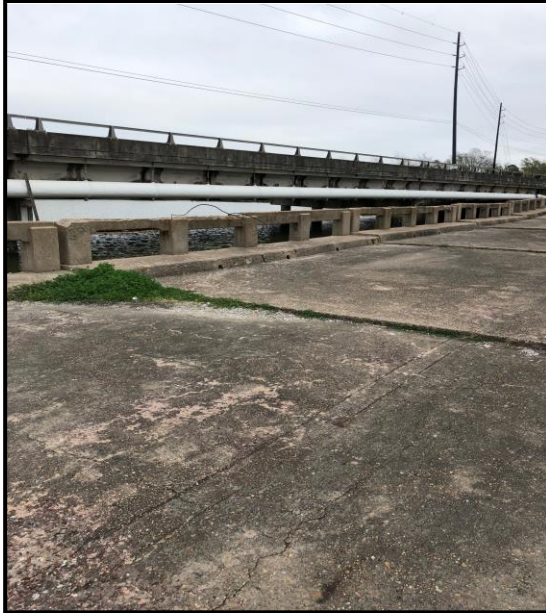
New bridge to allow for more freeboard
