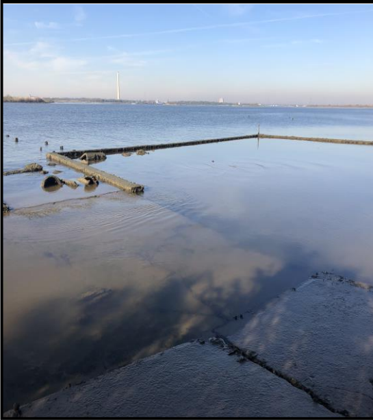
Home foundation remnants inundated
