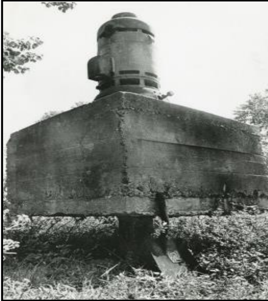
Reduced well capacity and casing damage
